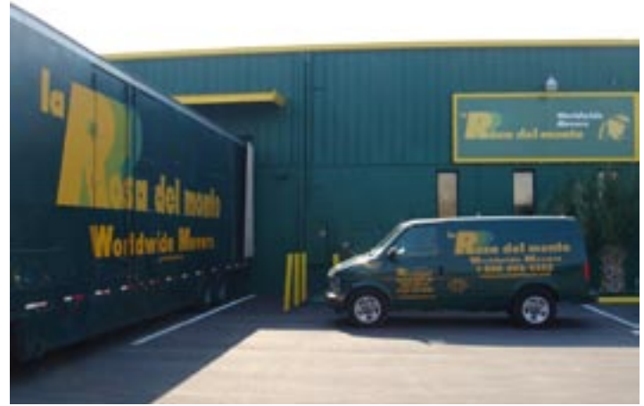
La Rosa Del Monte's facility in Orlando, Florida
