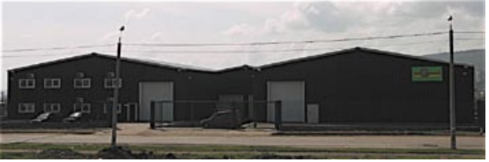
Gosselin's new custom-bonded warehouse in the Republic of Georgia.
