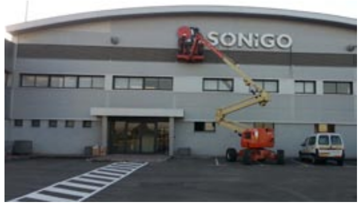
Sonigo makes its mark on its new facility.
